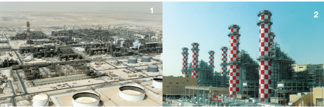
1. Pearl GTL project In November 2011, we completed EPC work on this advanced gas-to-liquids plant in Ras Laffan, Qatar. The plant is capable of producing 140,000 barrels a day of ultra-low-sulfur diesel, naphtha, LPG, and condensate using natural gas from undersea wells. 2. Al Dur independent water and power project In early 2012, we completed this turnkey EPC project for Al Dur Power and Water Company in Bahrain. The project includes a 1,245 MW combined-cycle power plant and 48 MIGD reverse osmosis desalination plant.
